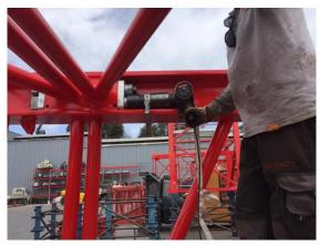
Figure 1: The angled electric torque multiplier ECWip100 from alkitronic on the crane bolting connection.
