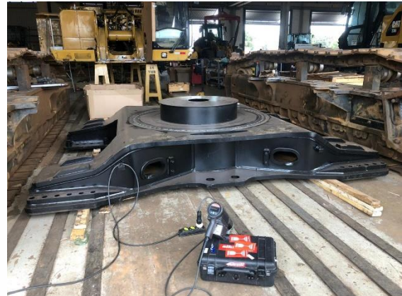
Figure 1: Large machines require reliable torque multipliers - picture: bolting on a turntable of a CAT excavator.
